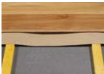
Tongue and groove planks can be secret nailed to a suitable existing timber subfloor.
