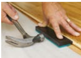
Floating a floor just means the boards are laid loose over the subfloor if they're a clic system, when floating a tongue & groove, the joints must be glued.
